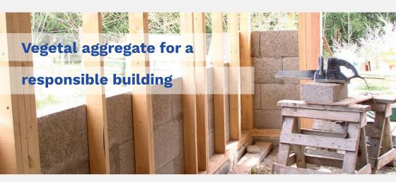
KANABAT, a plant-based aggregate, is derived from the mechanical processing of industrial hemp.
