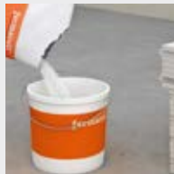
Figure 10: Add fermacell Joint Filler to water
