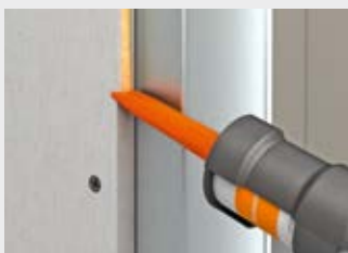
Figure 12: Guide the 310 ml cartridge along the edge of the board. The special nozzle releases the exact amount of adhesive for 10 and 12.5 mm boards. The nozzle must be cut for 15 and 18 mm boards.
