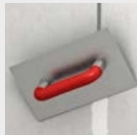
Figure 11: Fill joints and fixing heads
