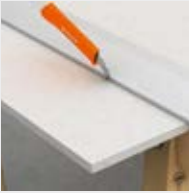
Figure 2: Measuring and scoring
