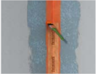
Figure 35: Press the fermacell Sealing Tape into the previously applied, wet fermacell Waterproofing Application and coat directly with the liquid waterproofing
