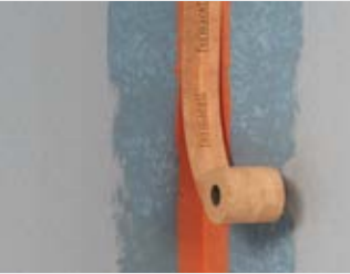
Figure 35: Press the fermacell Sealing Tape into the previously applied, wet fermacell Waterproofing Application and coat directly with the liquid waterproofing
