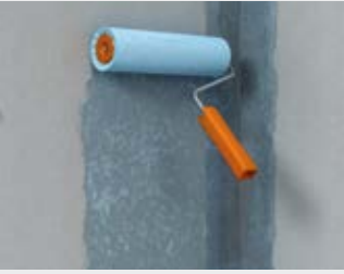
Figure 34: Full-surface application of fermacell Deep Primer
