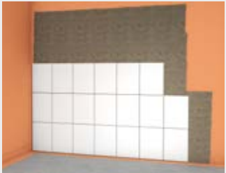
Figure 38: Tiling with fermacell Flexible Tile Adhesive depending on the moisture exposure class
