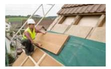
The ideal solution when the internal room finishes cannot be disturbed.
